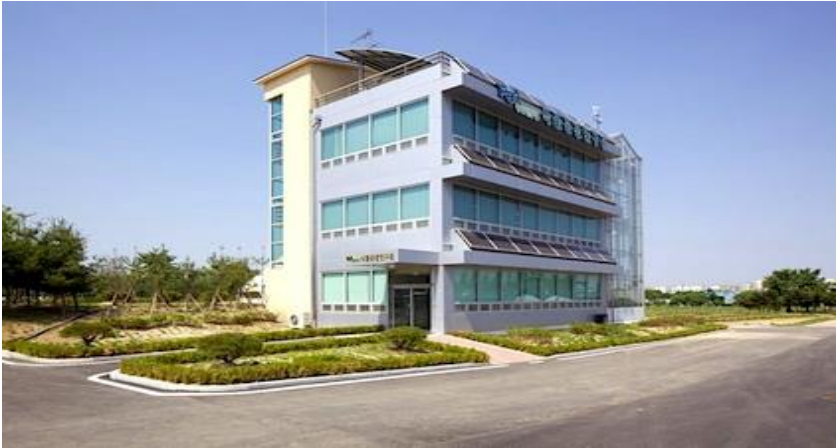
Figure 24: VF of Suwon, South Korea
