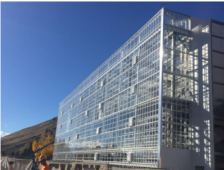
Figure 26: Project & construction of Vertical Harvest in Jackson, Wyoming
